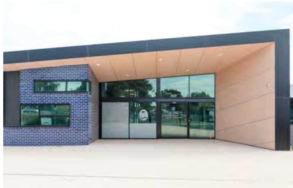
Hampton Park Primary School (rebuilt during 2017)
