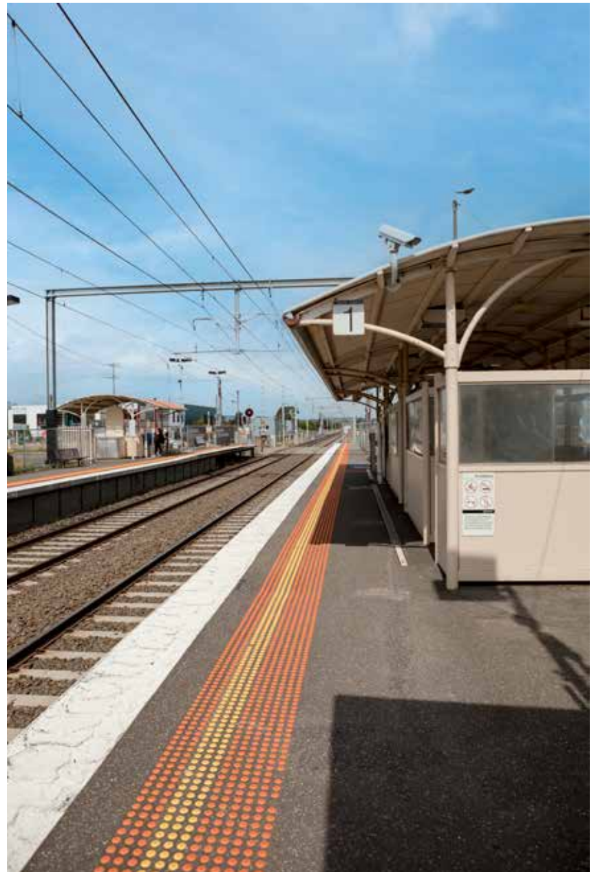
Hallam Station (To Be Revamped)
